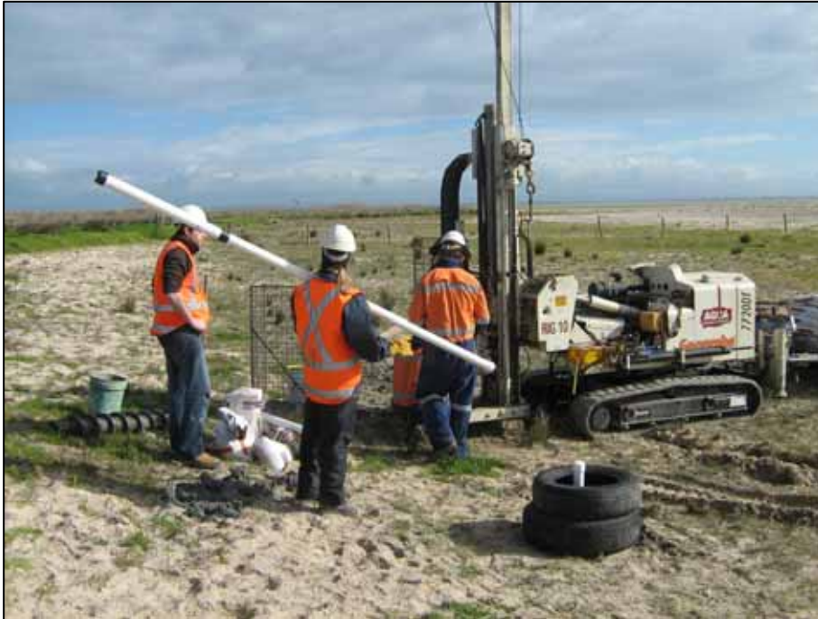
Plate 12. Piezometer installation at Campbell Park, Lake Albert.
