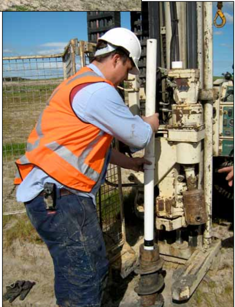
Plate 13. Hollow auger system used for piezometer installation. After inserting the piezometer to the required depth, the auger hole was backfilled with clean sand around the screened section and then capped with bentonite, whilst progressively removing the hollow auger rods.
