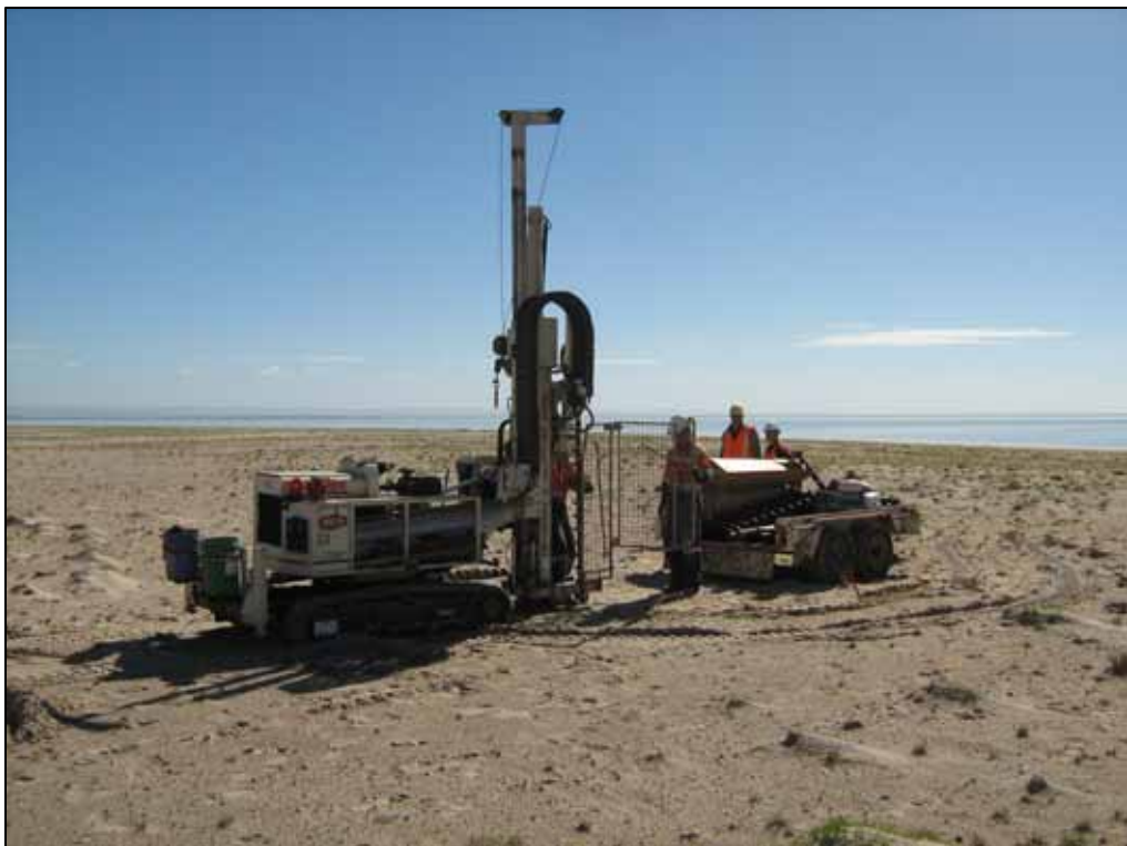
Plates 10-11. Geoprobe 7720DT drill rig used for sediment sampling and piezometer installation at Point Sturt (pictured), Campbell Park and Windmill locations.
